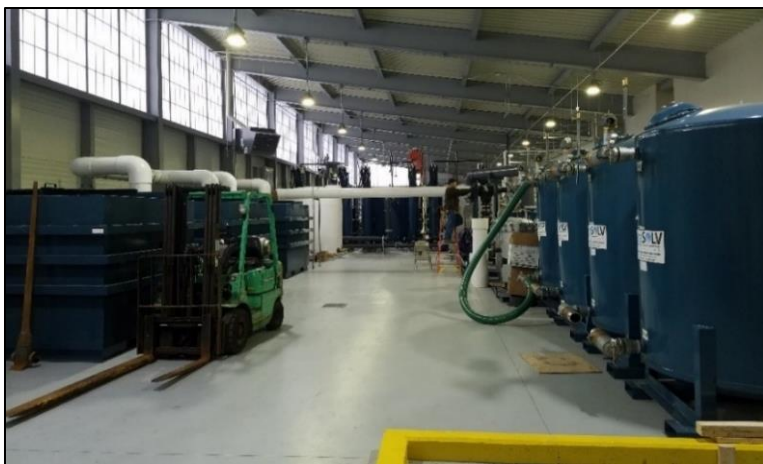
Groundwater treatment systems at the Southeast Rockford Groundwater Contamination National Priorities List site
