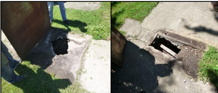
CDB is currently addressing deteriorating tunnel systems at the Shapiro Developmental Center.
