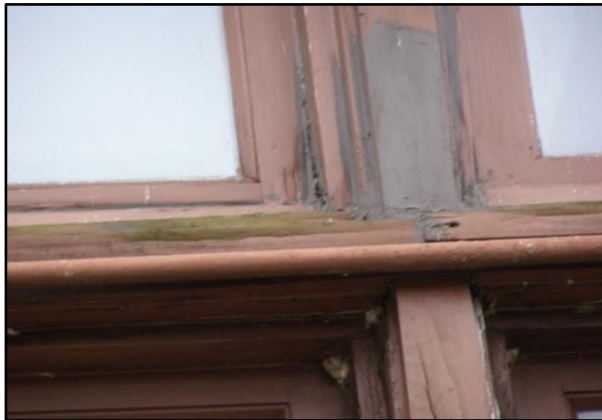
Close-up of damaged wood framing, found throughout the lodge, which will be replaced
