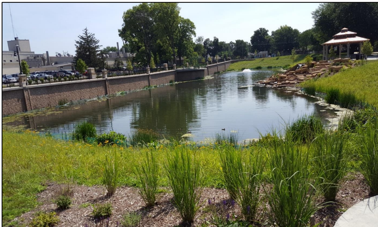
The City of Champaign's West Washington Street stormwater project incorporating green infrastructure to capture, control and treat stormwater
