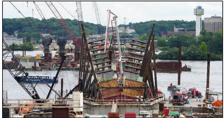
Construction at the I-74 bridge
