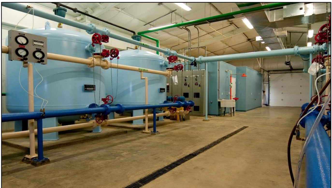
Water treatment plant control building in Winchester, Illinois
