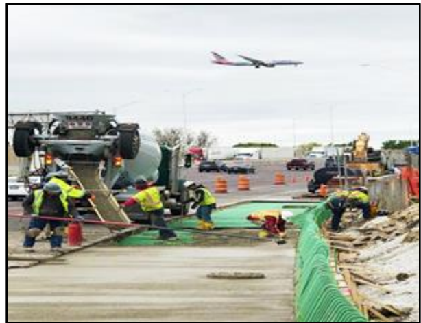
Reconstruction at Central Tri-State Tollway (I-294) near Rosemont
