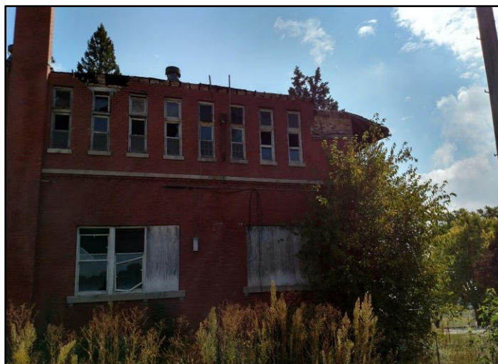
Harding Cottage at IYC St. Charles will be demolished
