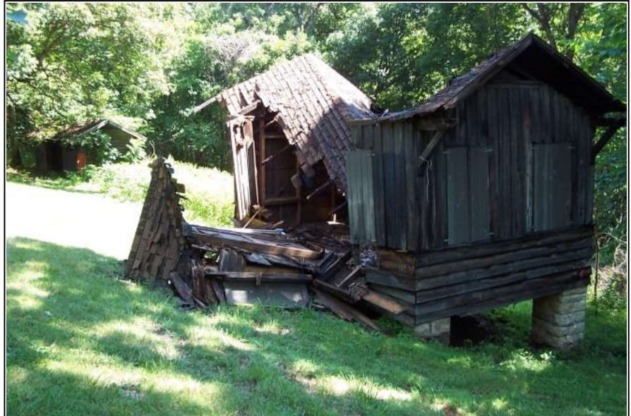
The tattered remains of a cabin at Pere Marquette State Park
