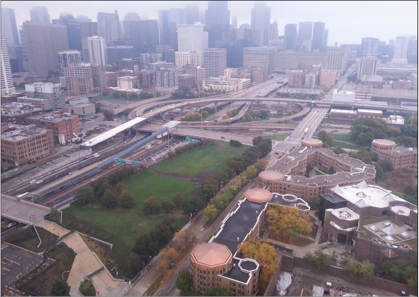
The Byrne Interchange under construction in October 2016. The ramp from the northbound Dan Ryan to the westbound Eisenhower, which opened in December 2016, is nearing completion above.
