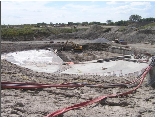
Construction of the base of the 1.5 million gallon first flush tank at the Riley Creek CSO Satellite Treatment Facility in the City of Mattoon
