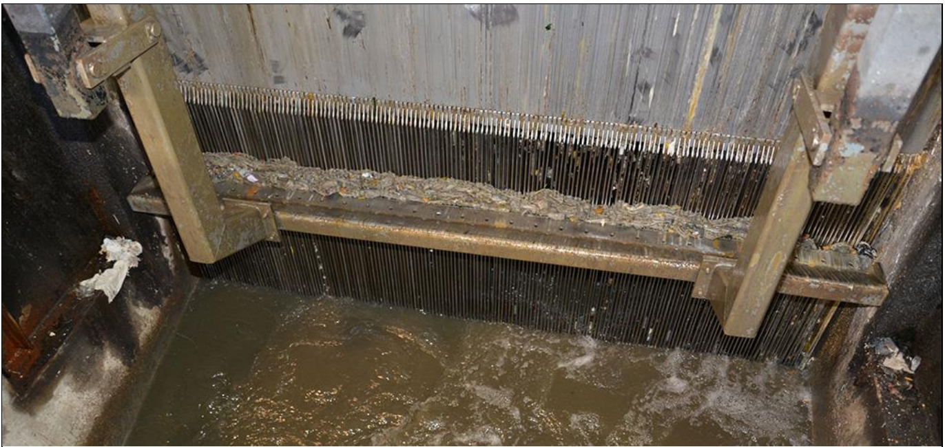
Raw sewage being filtered through bar filters at the Fox Metro Water Reclamation Plant
