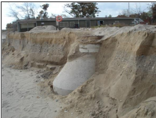
The exposed sewer line at Adeline Jay Geo-Karis Illinois Beach State Park
