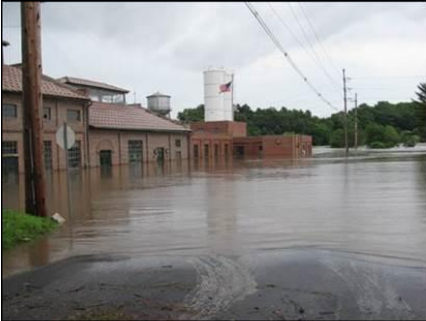
Flood damage to the former Jacksonville Water Treatment Plant in 2011
