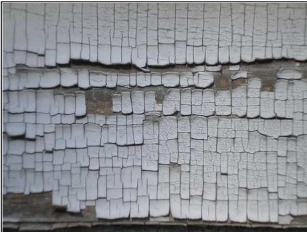
Though there is no substitute for testing for lead paint, it can sometimes be identified by a distinct square or rectangular shaped "alligator" pattern shown here.
