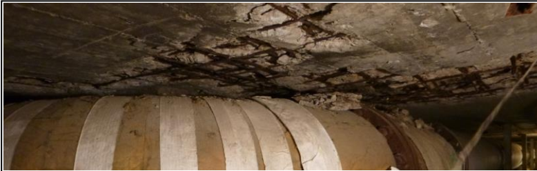
Severe spalling of the concrete roof of steam tunnels has caused roads above the tunnels to settle. Reports indicate that a car fell through a tunnel in 2015. Department of Human Services – Shapiro Mental Health Center – Kankakee
