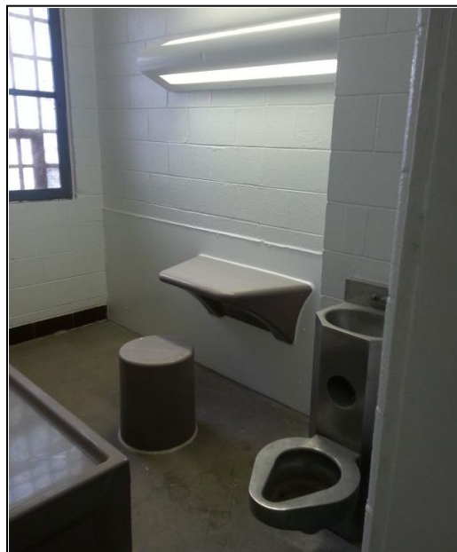
A nearly completed cell at JTC. Department of Corrections - Joliet Treatment Center - Joliet
