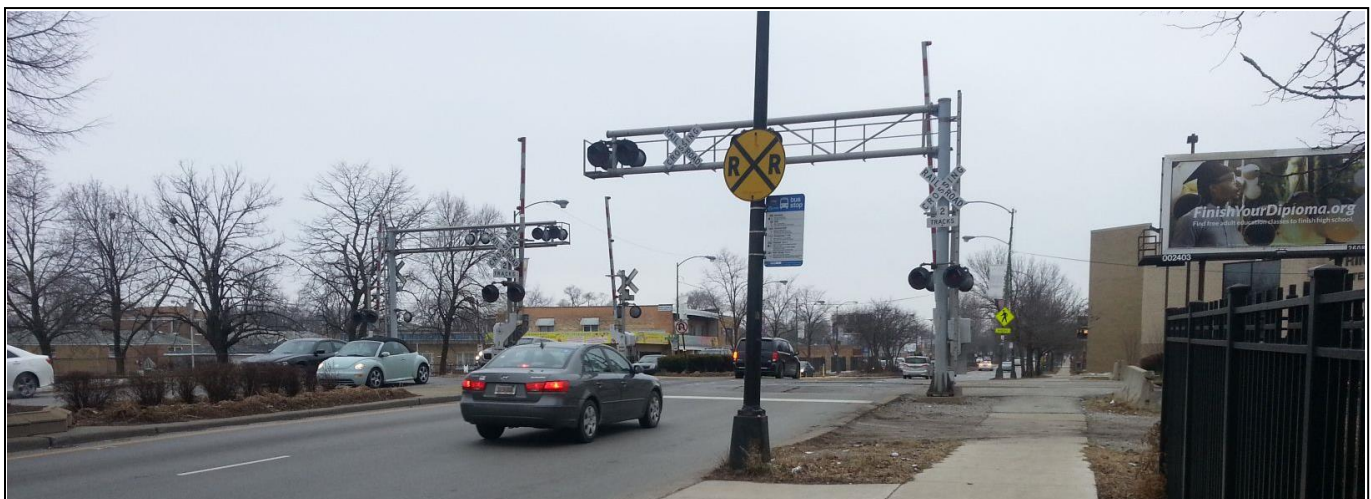
The Union Pacific grade crossing with 95 th Street in Chicago
