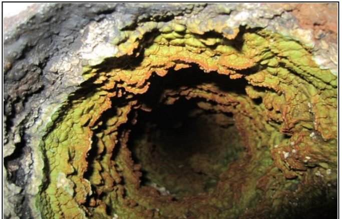
Below ground at the Capitol Complex, a pipe with a 50 percent blockage Secretary of State – Capitol Complex – Springfield
