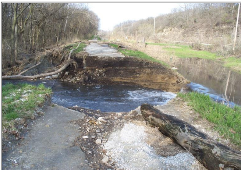
A washed out road at Illinois and Michigan Canal State Trail
