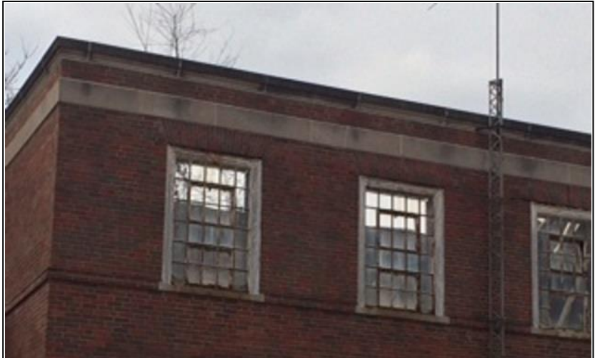
This building at Alton has a tree growing inside of it. The bright areas at the tops of the windows is the sky visible through the missing roof. Department of Human Services – Alton Mental Health Center – Alton
