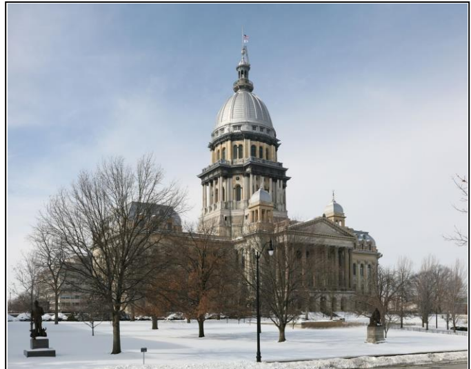
Above ground at the Capitol Complex Secretary of State – Capitol Complex – Springfield
