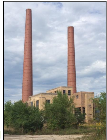
The power plant was built in 1900 and is well past its useful life. Department of Human Services – Elgin Mental Health Center – Elgin
