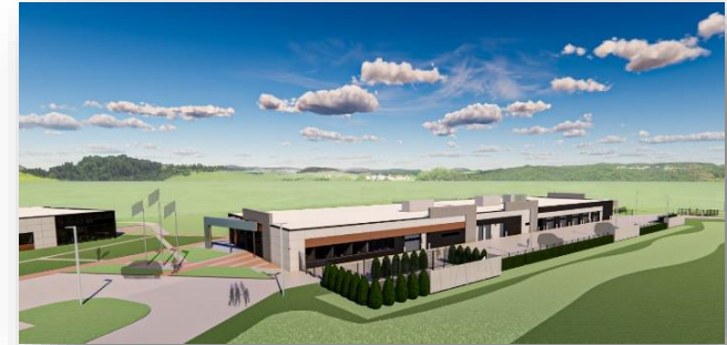
The design of the new ISP forensic lab in Joliet – one of the key projects from Rebuild Illinois
