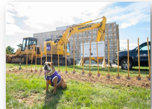
Construction Site at Western Illinois University Performing Arts Center
