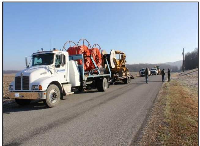
Truck carrying fiber and equipment
