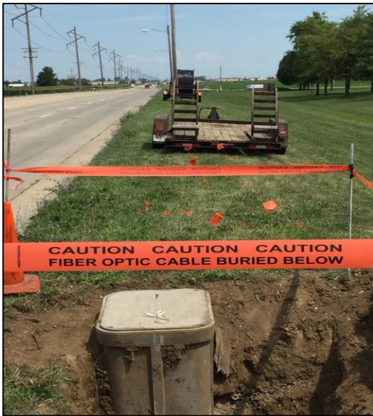
Decatur fiber project
