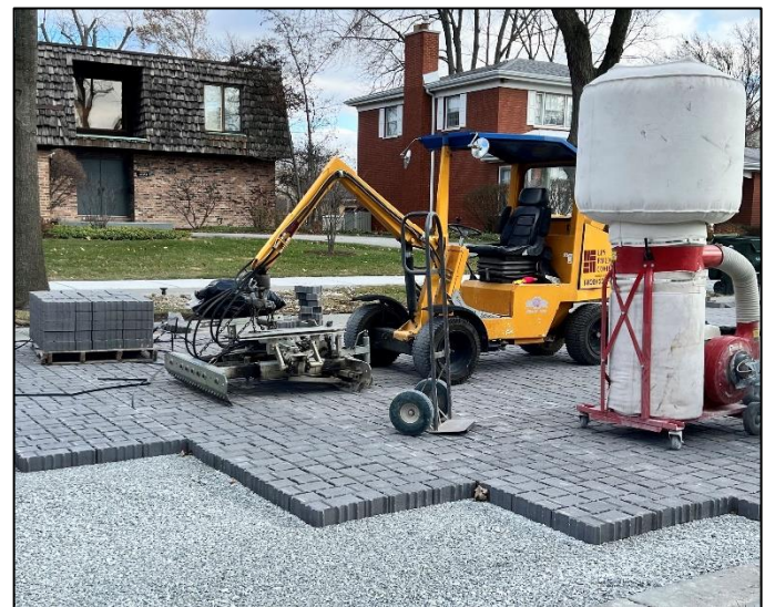
Porous Pavement installation at the Village of Flossmoor
