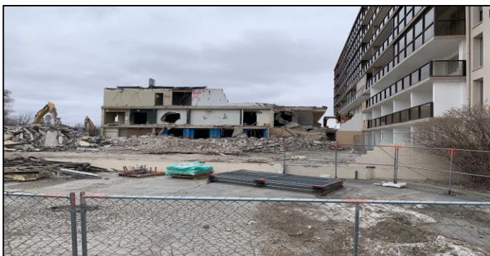
Progress during demolition, Rochelle
