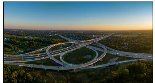
Completed I-294/I-57 interchange near Harvey, Markham, Dixmoor and Posen
