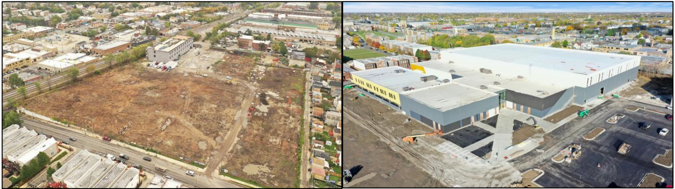
Future site and construction of the North Austin Community Center
