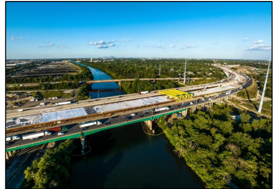
I-294 Southbound Mile Long Bridge Project near Willow Springs
