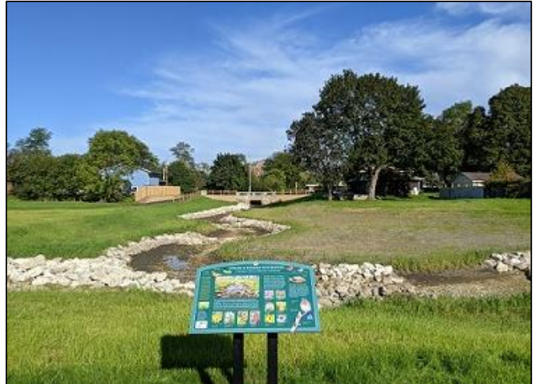
City of St. Charles – 7 th Avenue Creek Stream Restoration
