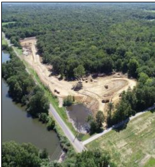
Forsythe Energy reclamation project near Cambria
