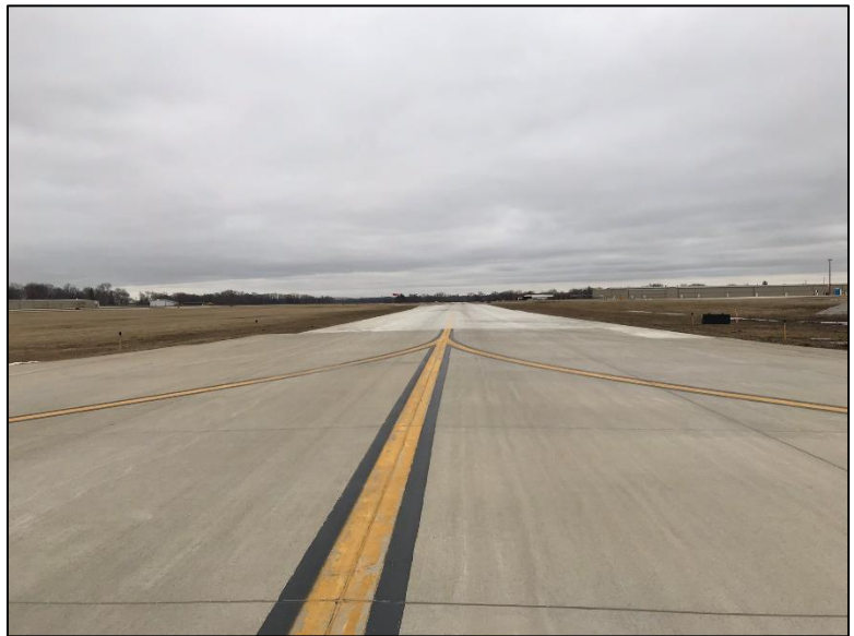
Lewis University Airport, Romeoville
