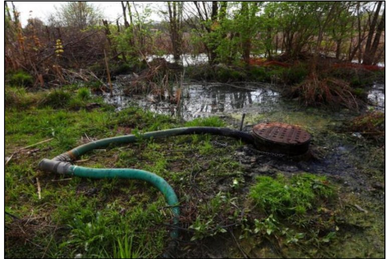
Cahokia Heights residential wastewater and sewage flooding
