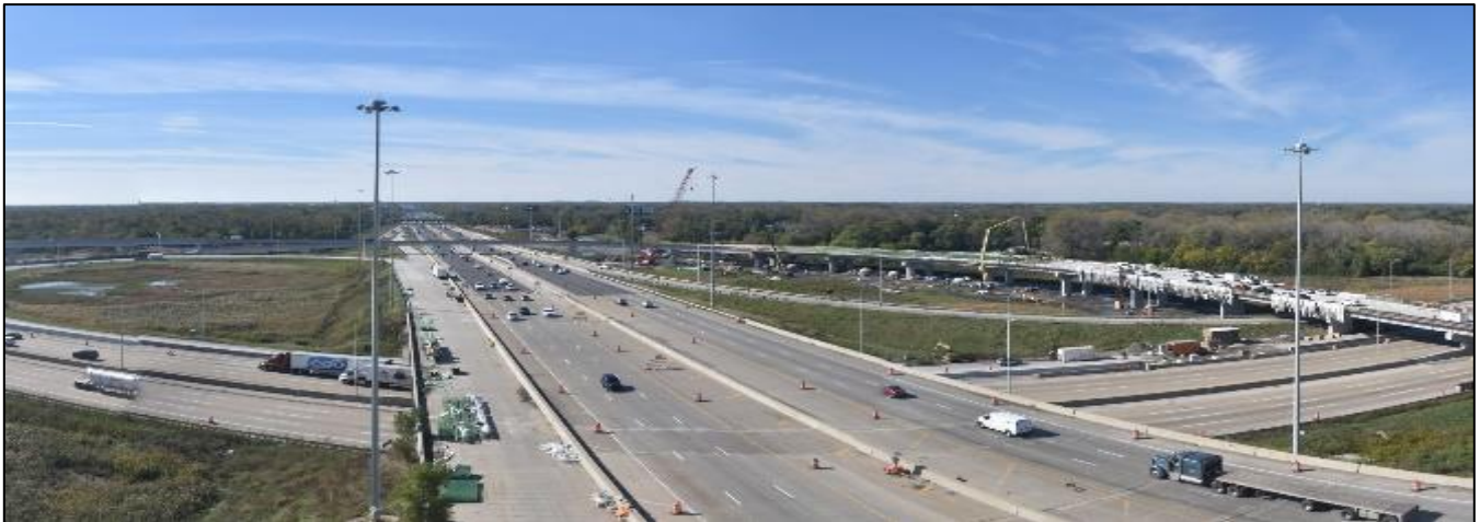
I-294/I-57 Interchange Project along the Central Tri-State Tollway (I-294) near Harvey
