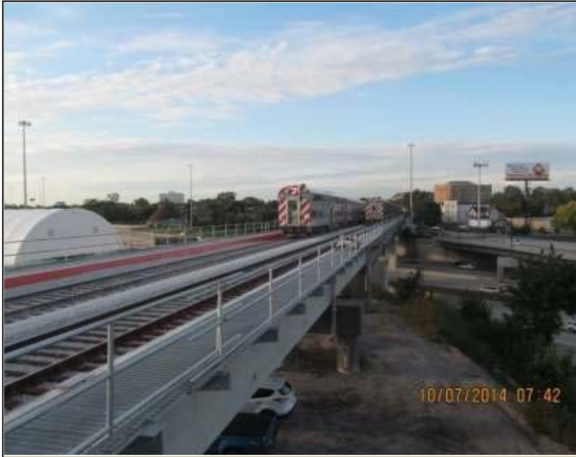
The Englewood Flyover, which saves 7,500 annual passenger hours of delay.
