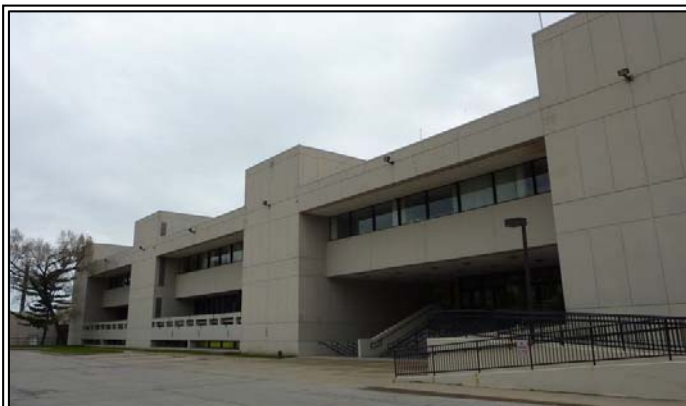
Department of Central Management Services – Maine North Regional Office Building – Des Plaines
