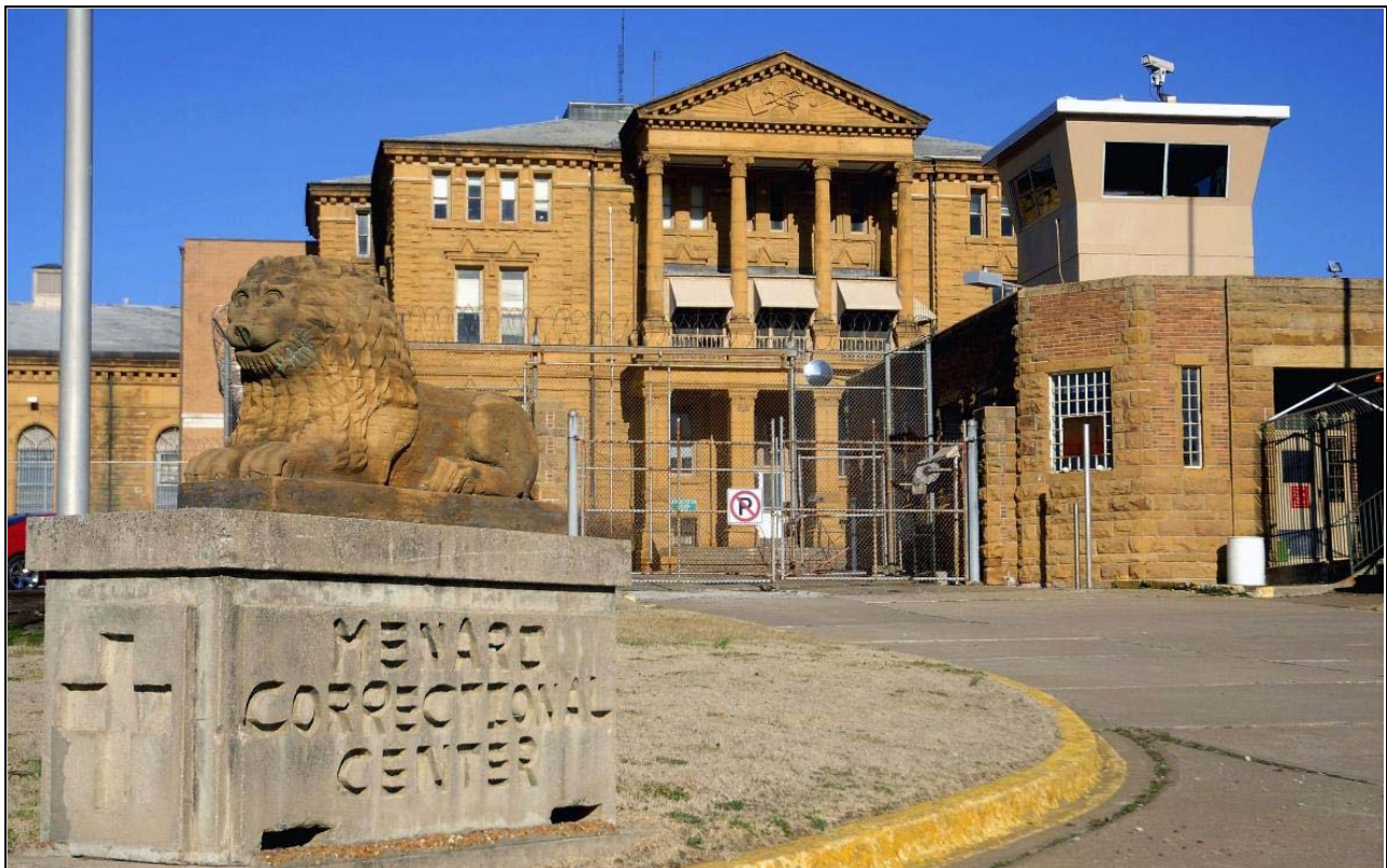
The Administration Building at Menard has been unable to fulfill its function for years and may be slated for demolition. Department of Corrections - Menard Correctional Center - Chester
