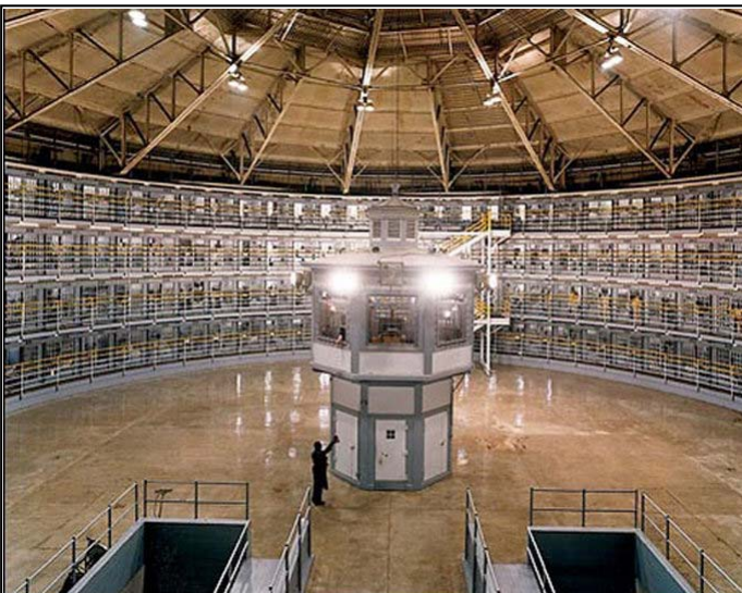
The interior of Cell House F, the “roundhouse”, one of many buildings at Stateville, the facility with the most deferred maintenance needs at DOC.
