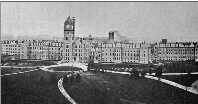
Shapiro Developmental Center, which opened in 1879, requires nearly $200 million in maintenance and has the most deferred maintenance needs of DHS' facilities.
