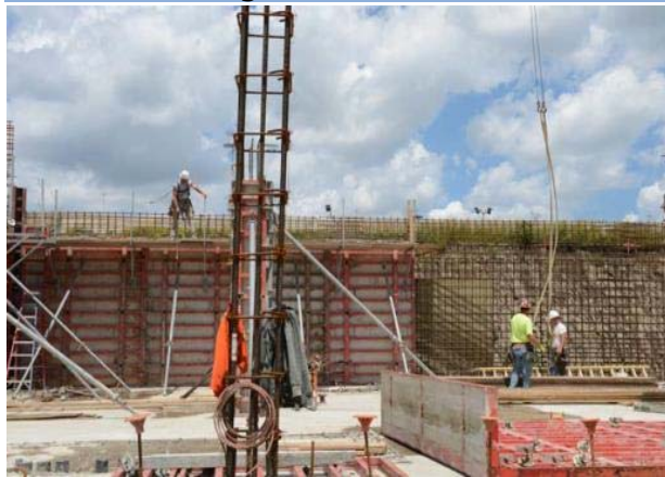
Calumet WRP Disinfection Construction
