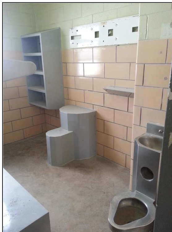
New anti-ligature and suicide resistant furnishings are being installed at IYC Joliet to ensure the safety of the inmates.
