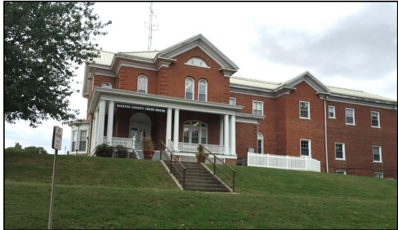
Mowing and grounds maintenance at Fayette County Courthouse and Jail Complex
