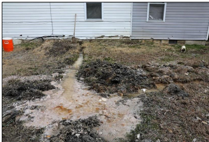
Centreville residential wastewater and sewage flooding
