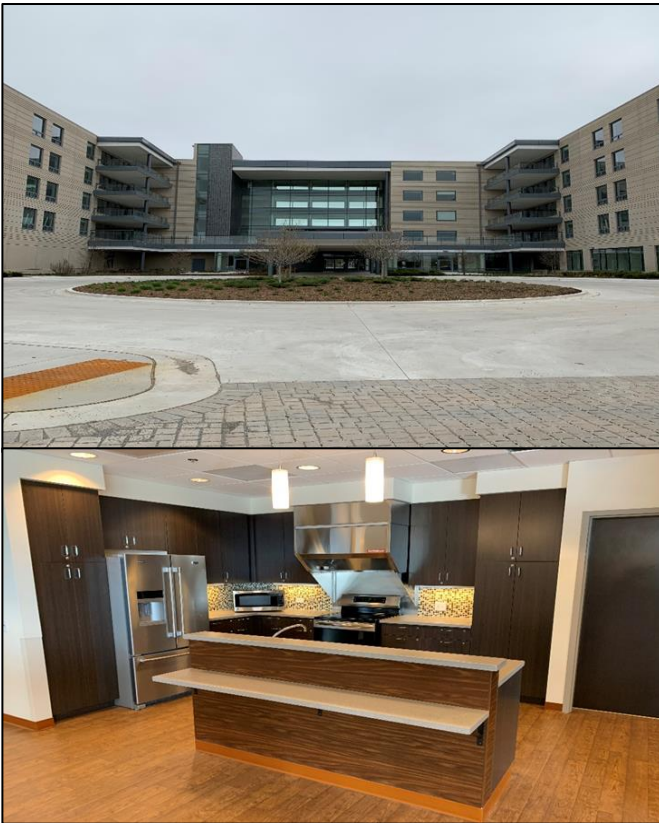
Top: South entrance of the Chicago Veterans' Home Bottom: Common area kitchen in the new home
