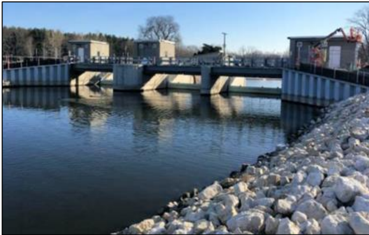
New Stratton Lock and Dam gate section
