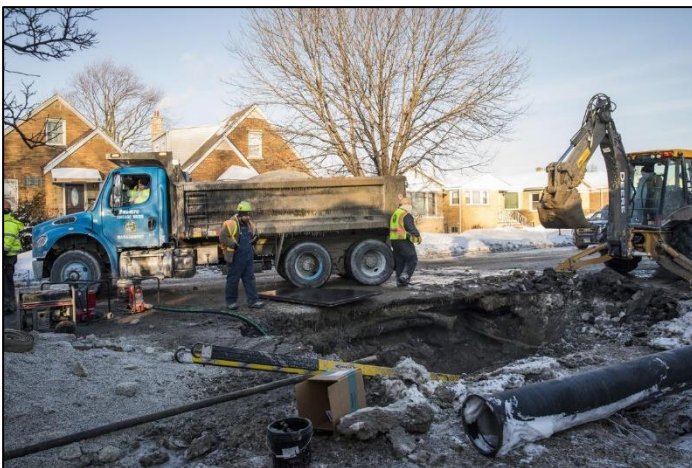
Lead service line replacement construction in Chicago
