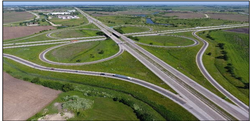
I-57/ I-74 Interchange
