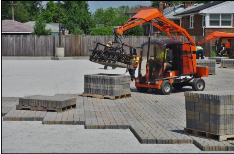
Installation of permeable pavers at Westchester Public Library
