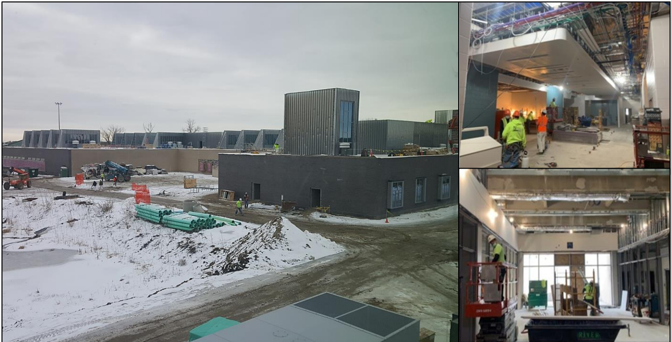
Joliet In-Patient Treatment Center under construction in January 2021
