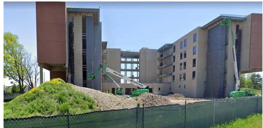
Chicago Veterans' Home under construction
